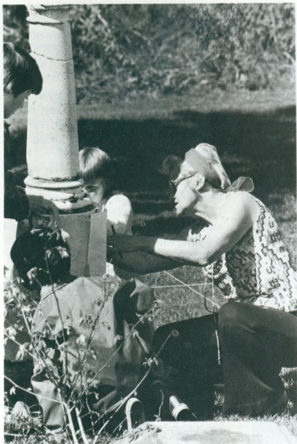
Leon Wootner, guided by Al Hummer, places a column on its pedestal after sealing cracks and cleaning the masonry (above).
