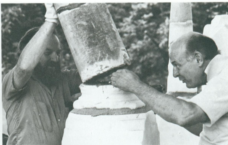
Leon Wootner, guided by Al Hummer, places a column on its pedestal after sealing cracks and cleaning the masonry (above).
